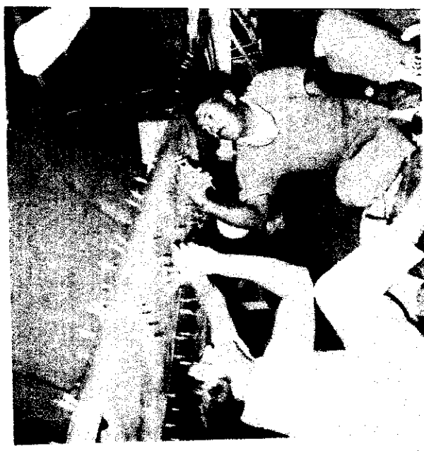
Finishing Landing Edge of Wing
